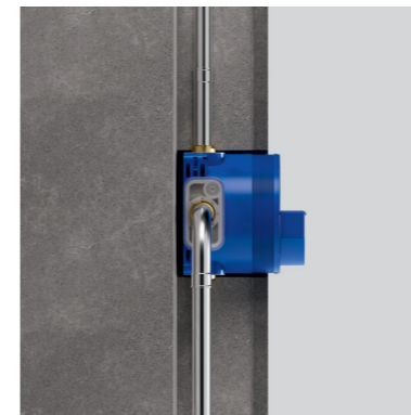
Installation in the wall
