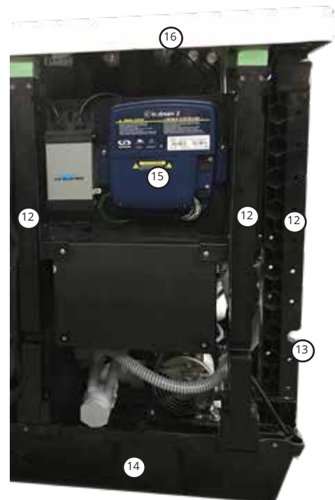
Corner Compartment (left front)
